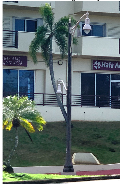
D. Streetlight & Sidewalk Light
